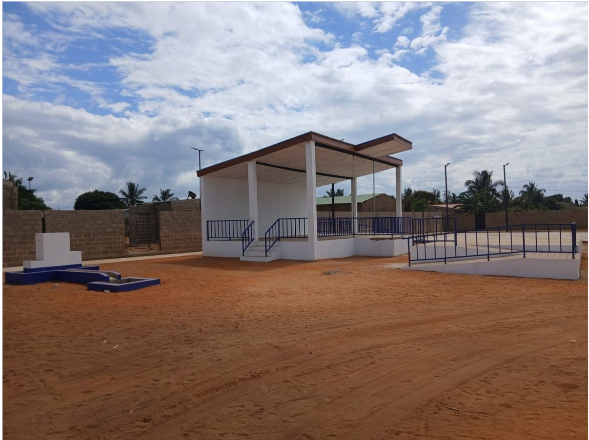
The Muxara public space taking shape, with the covered pavilion and the multi-use fields beyond.
