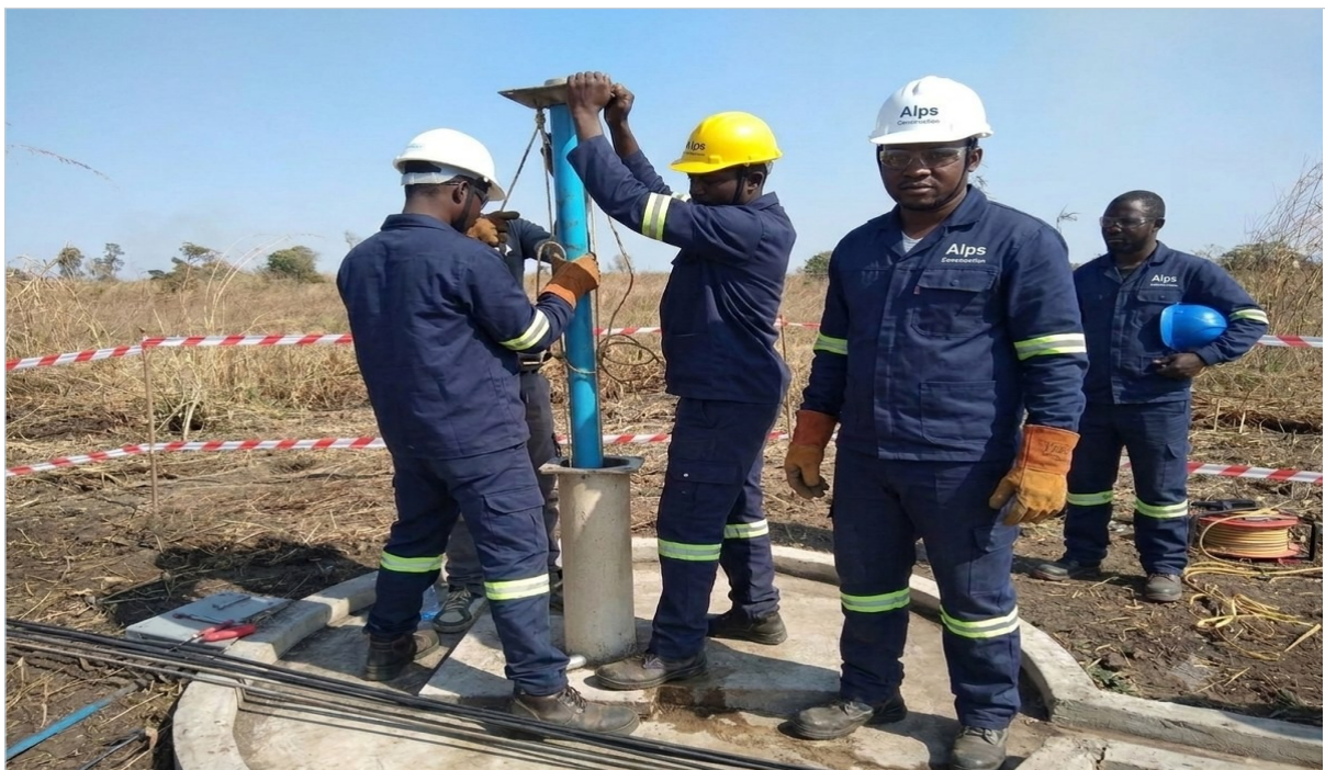
ALPS Constructions technicians rehabilitating an Afridev handpump in Chiure district.
